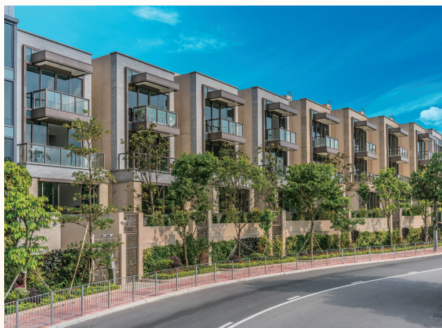
Exterior view of the garden houses at Casa Regalia
