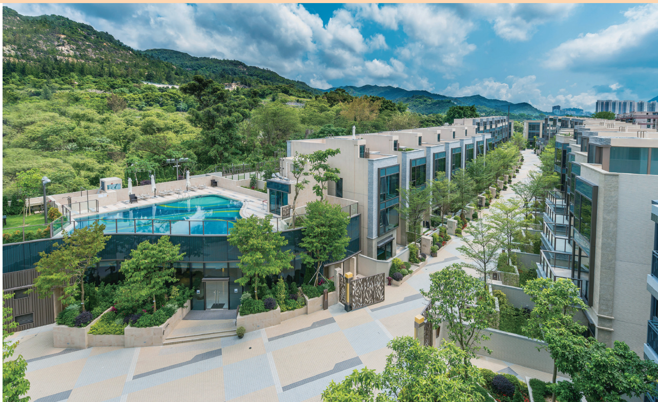
Casa Regalia, the garden houses in the residential development at Nos. 65-89 Tan Kwai Tsuen Road, Yuen Long, New Territories
