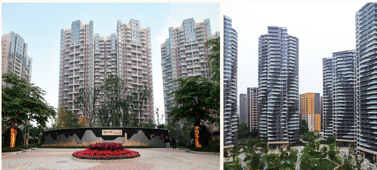
Casa Regalia (Phase 1 and Phase 2) - residential component of Regal Cosmopolitan City
