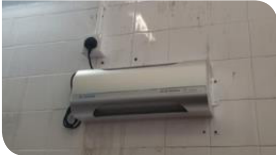
UV air sterilisation device for garbage room
