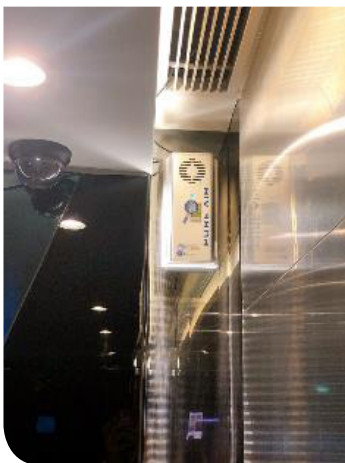
UV air purifiers in the lift
