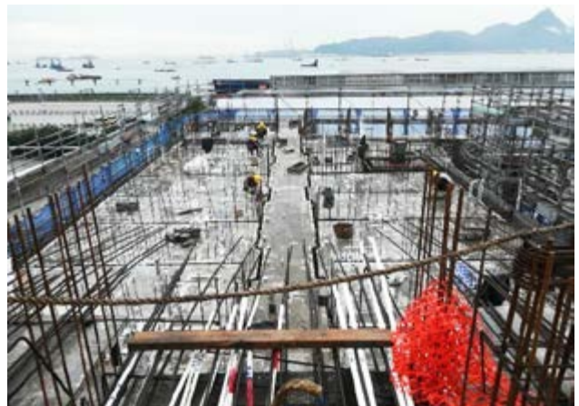
Aluminium formwork is used for the construction of typical floors to reduce timber use.
