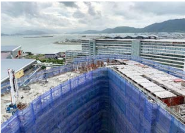
Aluminium formwork is used for the construction of typical floors to reduce timber use.
