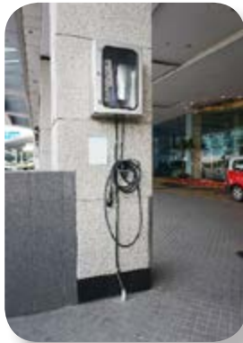
Electric vehicle charging station at Regal Airport Hotel
