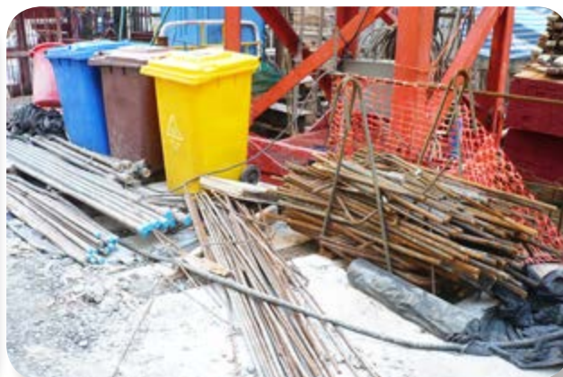
On site waste sorting area
