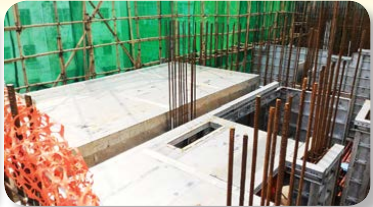
Aluminum formwork are used for the construction of typical floors to reduce timber use
