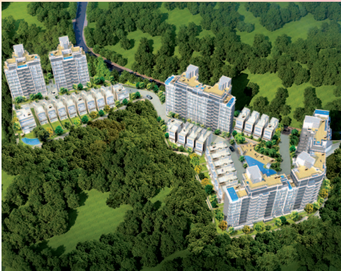
■ Luxurious residential development at Sha Tin Town Lot No. 578, Area 56A, Kau To, Sha Tin, New Territories – foundation works in progress (*)
